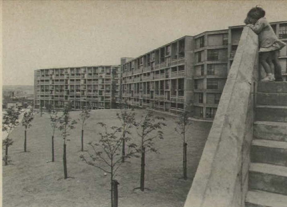
Park Hill Apartments, Sheffield, England.
